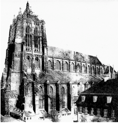
7-6 Ulm Minster, 19th-century photo showing flanges on wall where flying buttresses would be installed.
