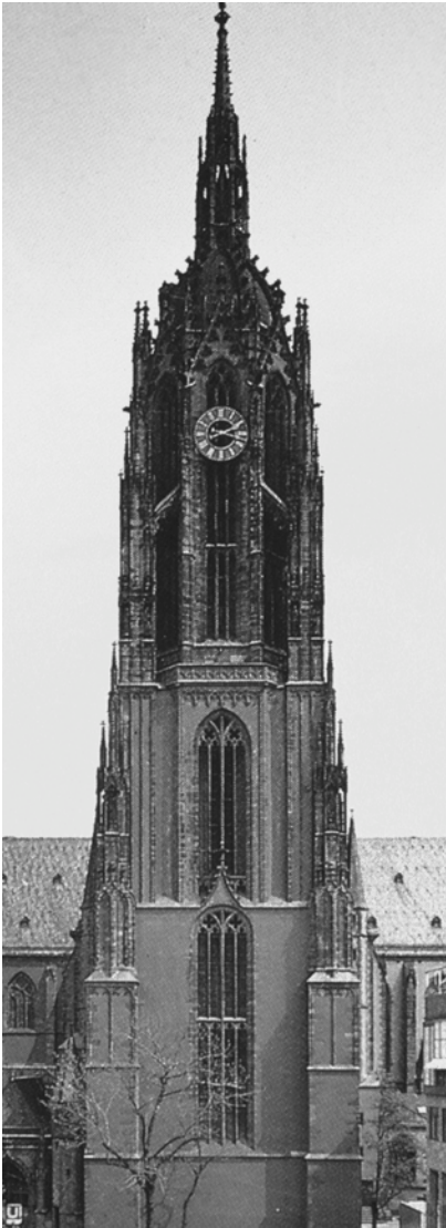
8-19 Frankfurt, St. Bartholomäus, view of tower from west.
