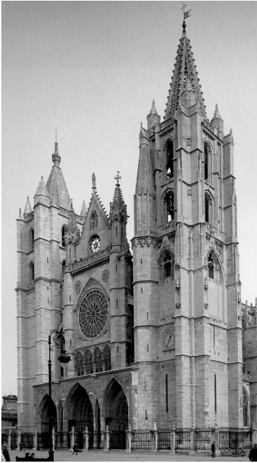
9-21 León Cathedral, west facade.
