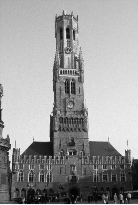
9-2 Bruges, market hall.
