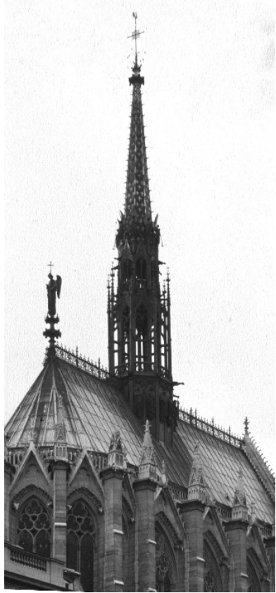
10-2 Paris, the Sainte-Chapelle, roof and spire.
