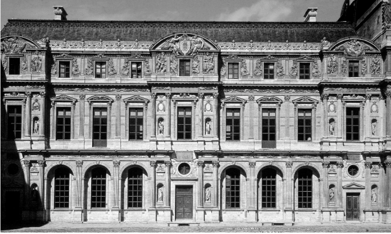
11-2 Paris, the Louvre, facade of Square Court.
