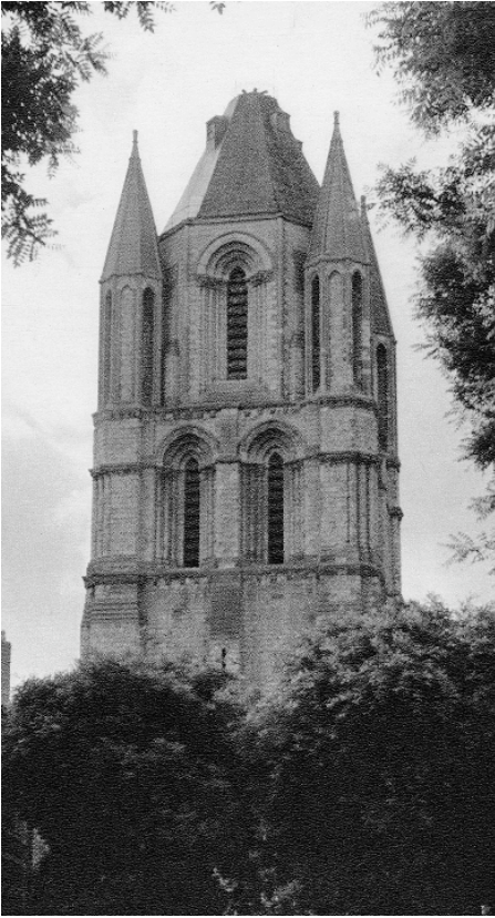
2-7 Angers, Saint-Aubin, tower.
